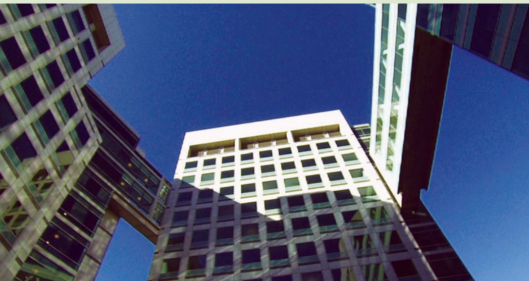
Sky bridges between towers © William Porter
