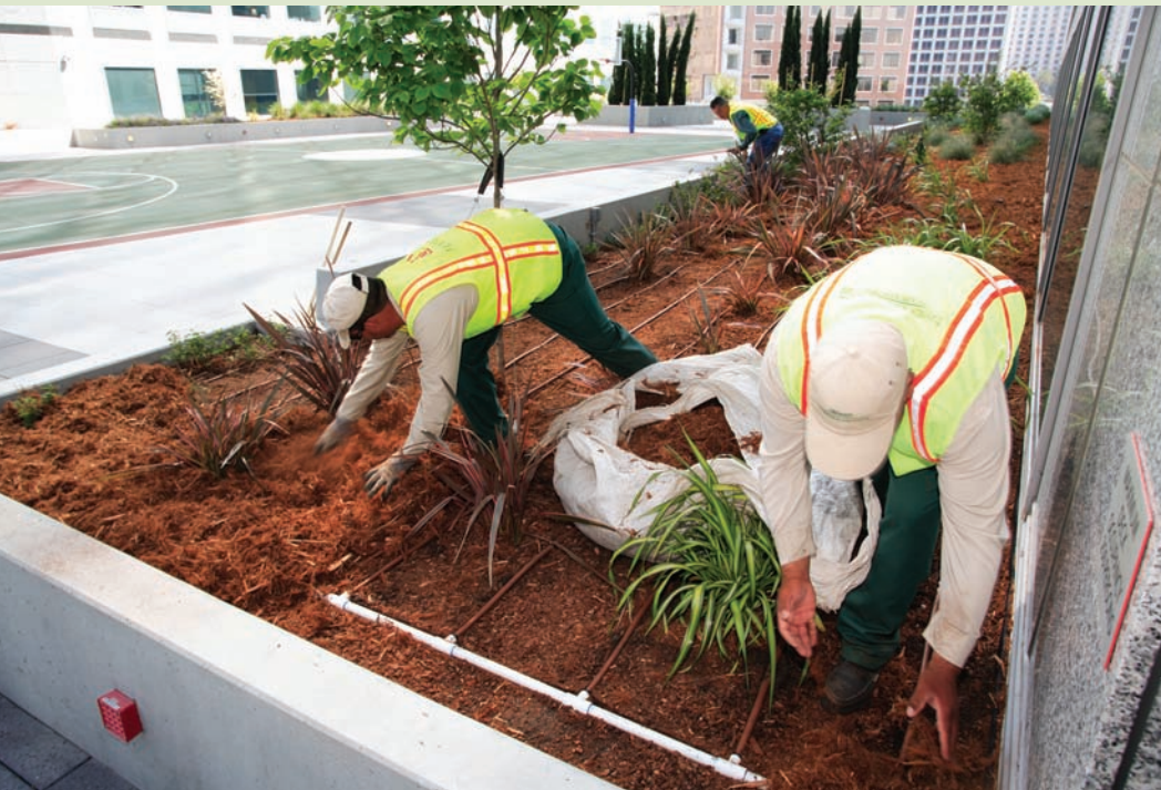
Installation of drip irrigation system / © William Porter
