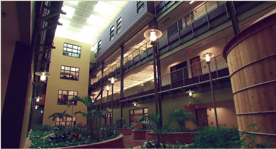
Rainwater cistern in atrium / © Jim Schafer Location Photography
