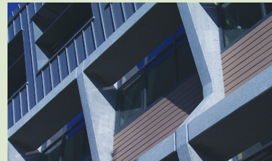
Detail of concrete overhangs and fins © Rocky Mountain Institute
