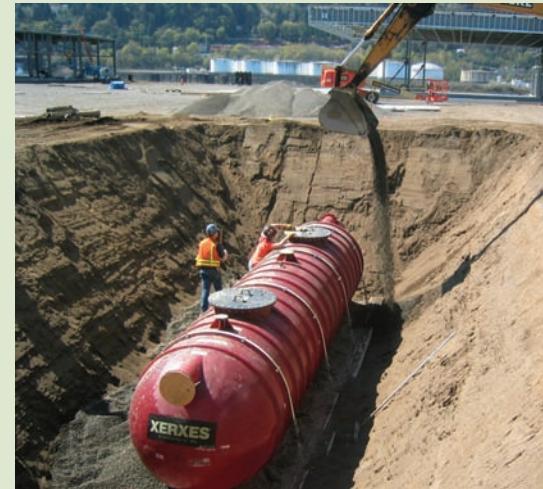
Installation of rainwater-harvesting storage tank / © Toyota Motor Sales, USA, Inc.
